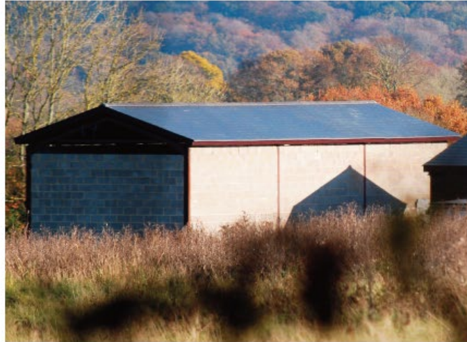
West view from woodland - illustrating brand new slate roof
