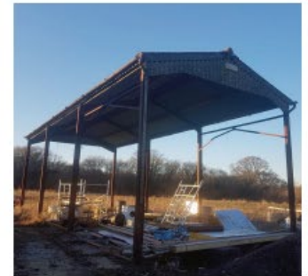
Original barn before development showing original asbestos/concrete style roof
