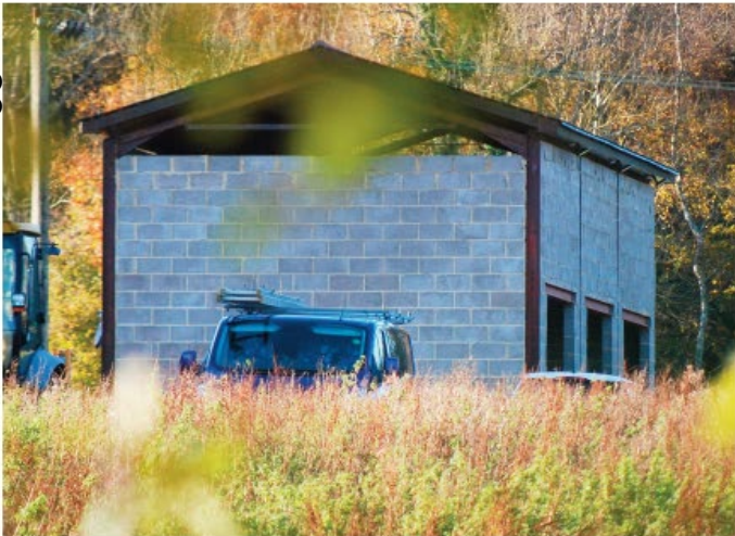
North East view from adjoining farmland (with permission) illustrating block work, plus three large openings, and new guttering.
